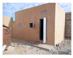
steady temperature of around 64 degrees F. Next, bottle walls are said to be 20 times stronger than concrete cinder blocks. The job of filling the bottles with sand can be given to people without jobs and even to the handicapped. And finally, non-degradable plastic bottles can be used for something constructive as opposed to filling our landfills and oceans.
