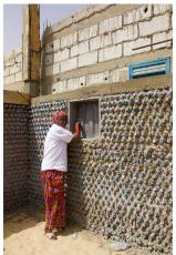
They are collected from hotels, restaurants, embassies, and, of course, local landfills. They are filled with sand, which is abundant, and packed as tightly as possible. Then they are used in just the same way bricks are, with mortar and string lines to keep everything level. After the walls are built and the roof put on (often a tin roof)
